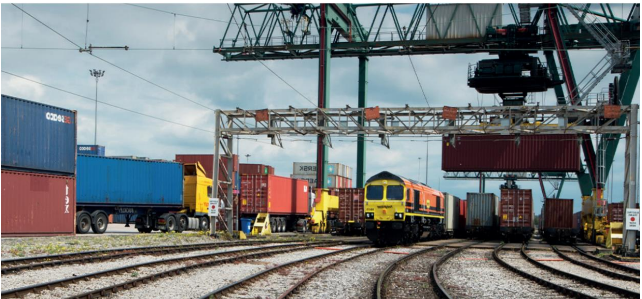
Figure 2 Rail Mounted Gantry Crane (RTG)
