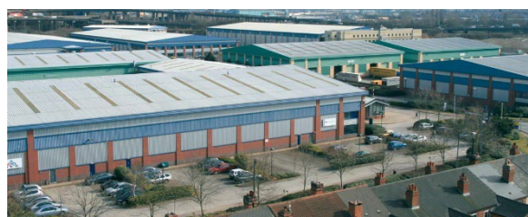
Junction 6 Electric Avenue, Birmingham - Prime urban logistics three miles from centre of Birmingham. Acquired off-market in July 2023.
