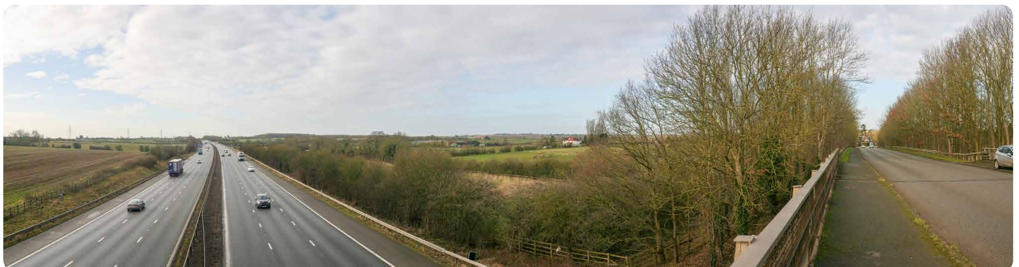
■ View looking south west towards site from B581 Station Road bridge over M69
