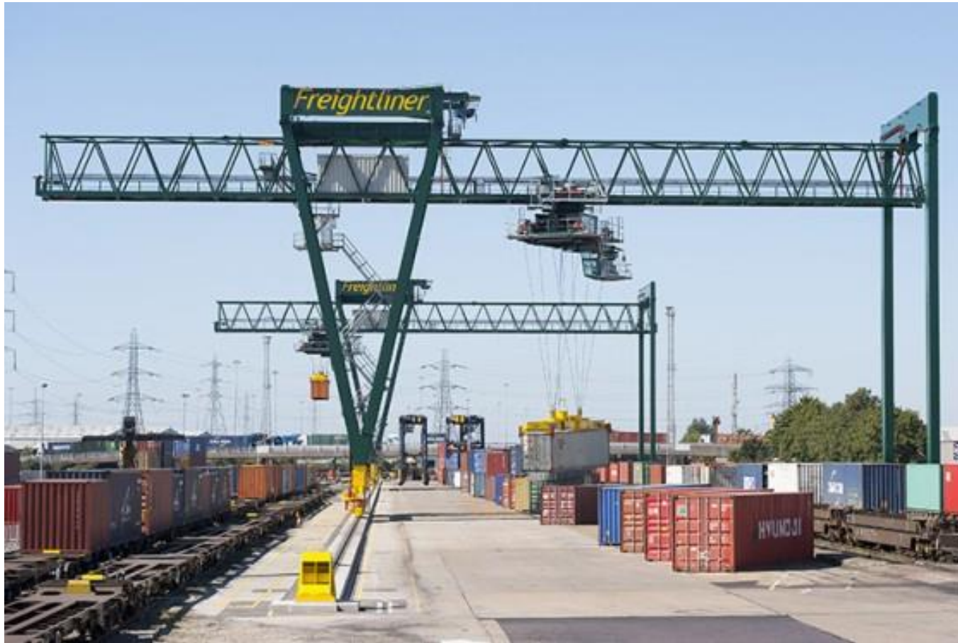
Figure 5-2 - Gantry Cranes Operating in a Uk Railport
